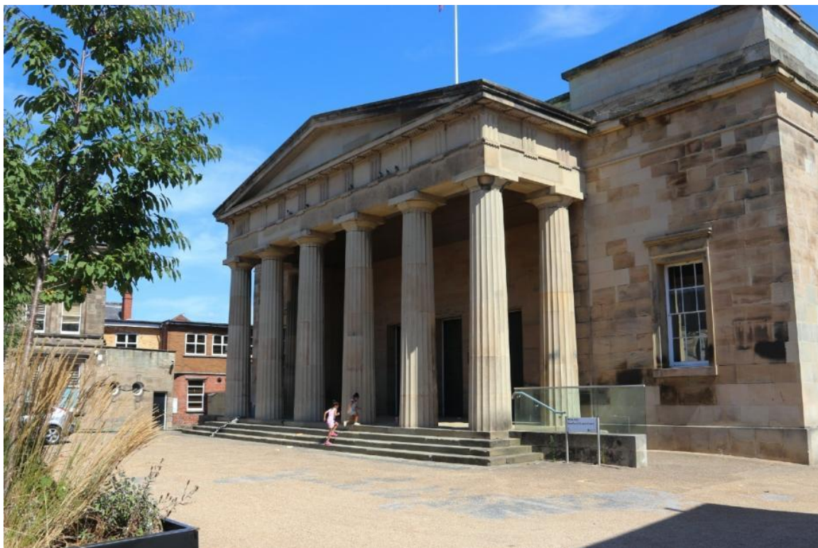
Fig 11: Front of Shirehall building
